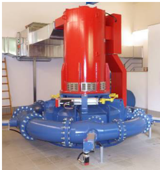
Pelton turbine/Generator
